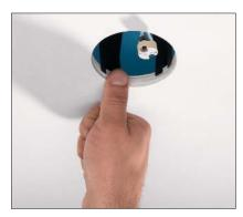
Push the retaining spikes into the plasterboard to prevent subsequent shifting.
