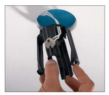
Fix the supply cable in place, push the mounting clips together, and insert in the ceiling cavity.
