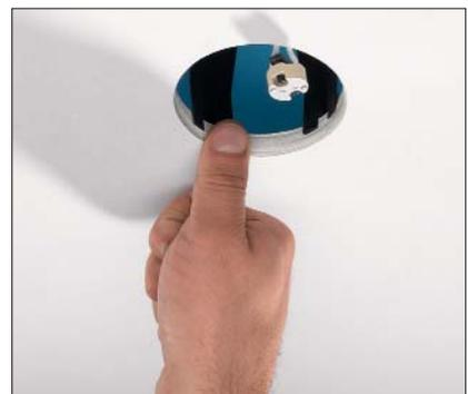
Push the retaining spikes into the plasterboard to prevent subsequent shifting.
