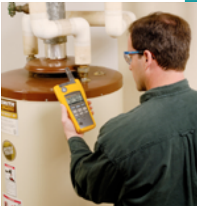
Technician using the 975 AirMeter to check for carbon monoxide leaks.
