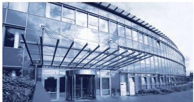
Basler AG Germany, Headquarters
