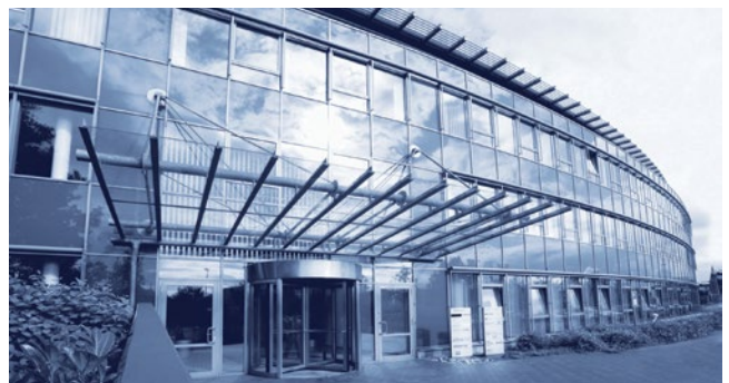
Basler AG Germany, Headquarters
