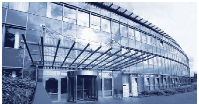
Basler AG Germany, Headquarters
