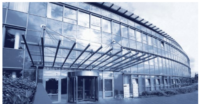
Basler AG Germany, Headquarters
