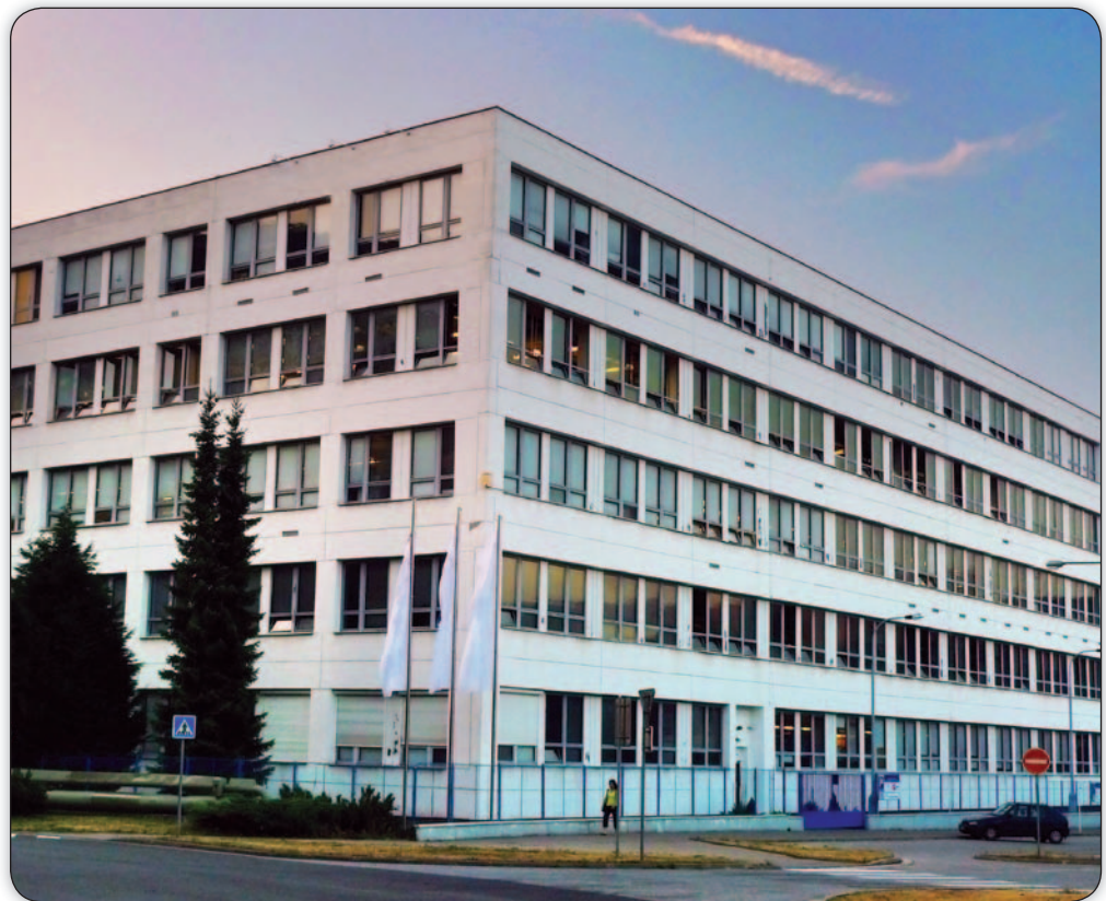
TE Manufacturing Facility in Trutnov, Czech Republic
