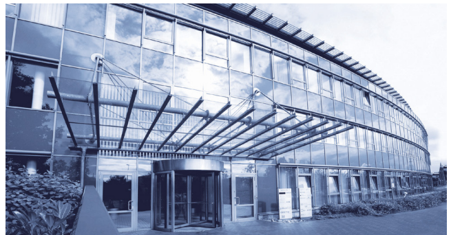
Basler AG Germany, Headquarters
